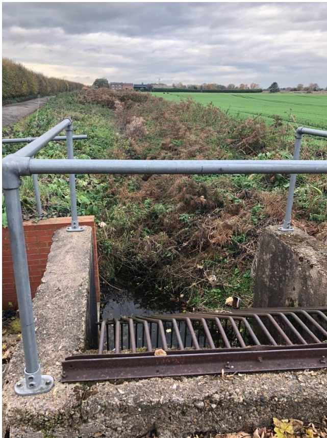
PHOTO 10: VIEW NW UP ROSCOE ROAD – END OF FIELD DRAIN ENTERING CULVERT
